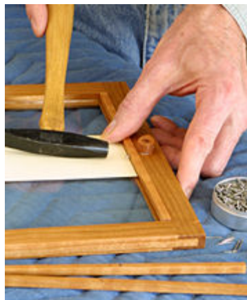
After the glass is set into the rabbet, small glass supports are nailed into place.
